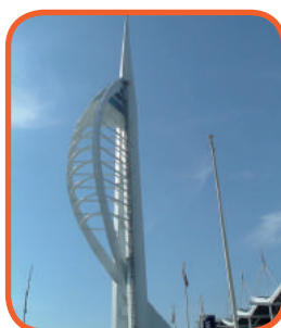
Portsmouth - Spinnaker Tower
